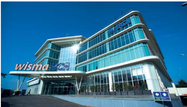
BCA builds its office buildings based on the energy saving and environment-friendly principles.
