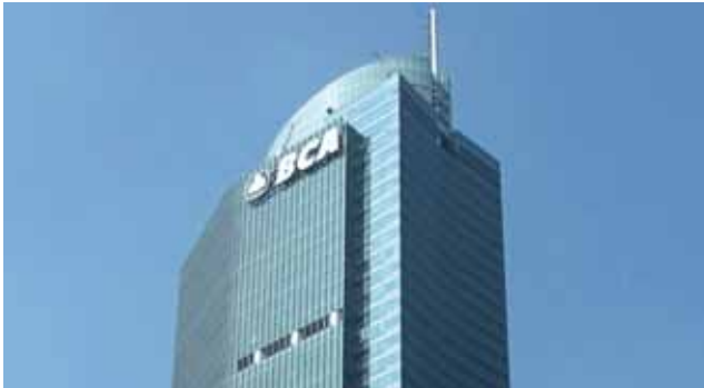
BCA Tower, the first building in Indonesia to receive the GREENSHIP EB Platinum.
